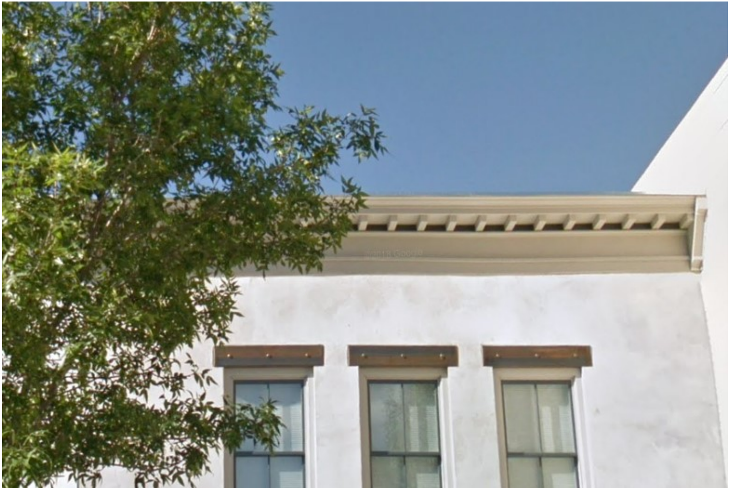
(3.3.2) Where a flat roof is appropriate on a commercial or mixed use building (as outlined above) and is used, design it to be screened from view.
