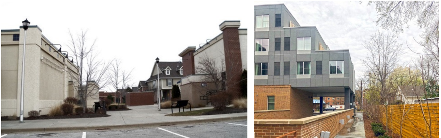
(2.3.1) Mitigate negative impacts of a large building on a sensitive property. The left image does not illustrate an upper floor setback to the residential use. However, the right image illustrates stepping a building's height down toward the sensitive use, residential in this case.
