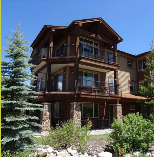
These guidelines promote a cohesive development pattern, while allowing for a level of diversity and creativity in the design and construction of individual projects.
