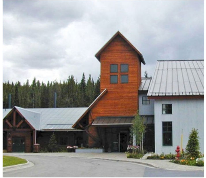
(3.7.2) Mass variation reduces actual building mass and scale by modulating building volume.
