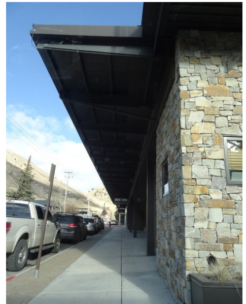
(3.3.8) Incorporate deep eaves, overhangs, canopies, and other building features that provide shelter from the elements.
