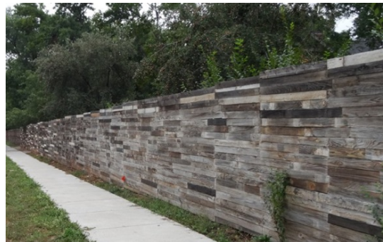
(2.6.2) Vary design elements to enhance visual interest and provide a sense of scale.
