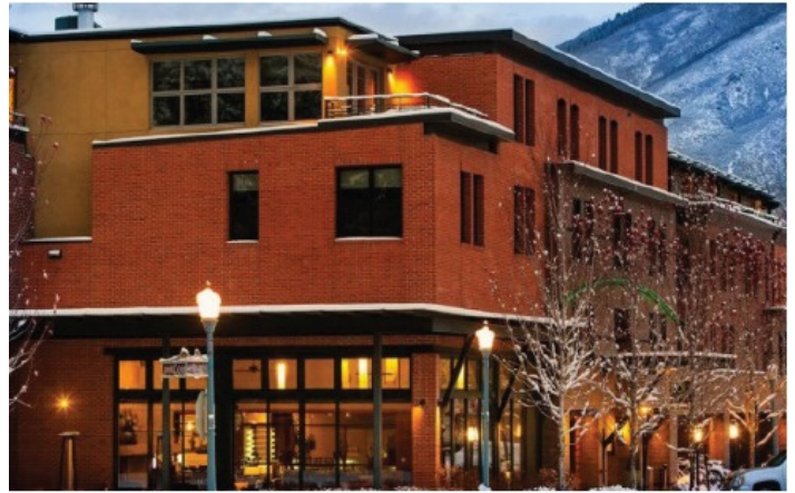
(3.7.1) Wall plane offsets articulate a building wall to create human scale components.
