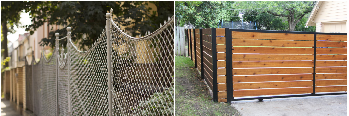
(2.6.3) Use a material that is durable and compatible with that of adjacent buildings and other site features. The chain link fence is inappropriate, while the cedar fence to the right is appropriate.
