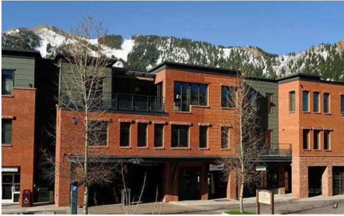
(3.7.1) Articulate a building wall to create human scale components and express a sense of vertical and horizontal scale.
