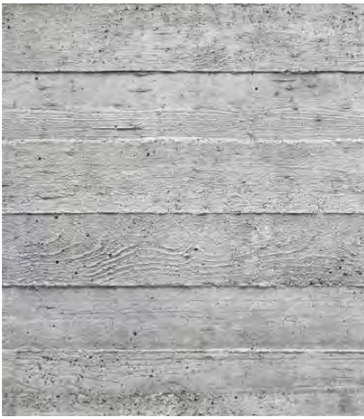
BOARD-FORMED CONCRETE FINISH (8" FORMS) (BELOW EAST TERRACE & MAIN LEVEL RESTROOMS - WEST SIDE)
