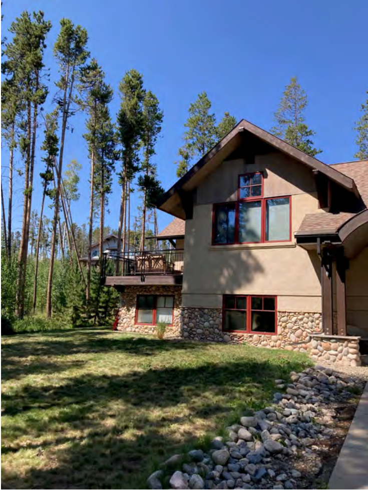
Existing Site Photos: 07.31.2024
