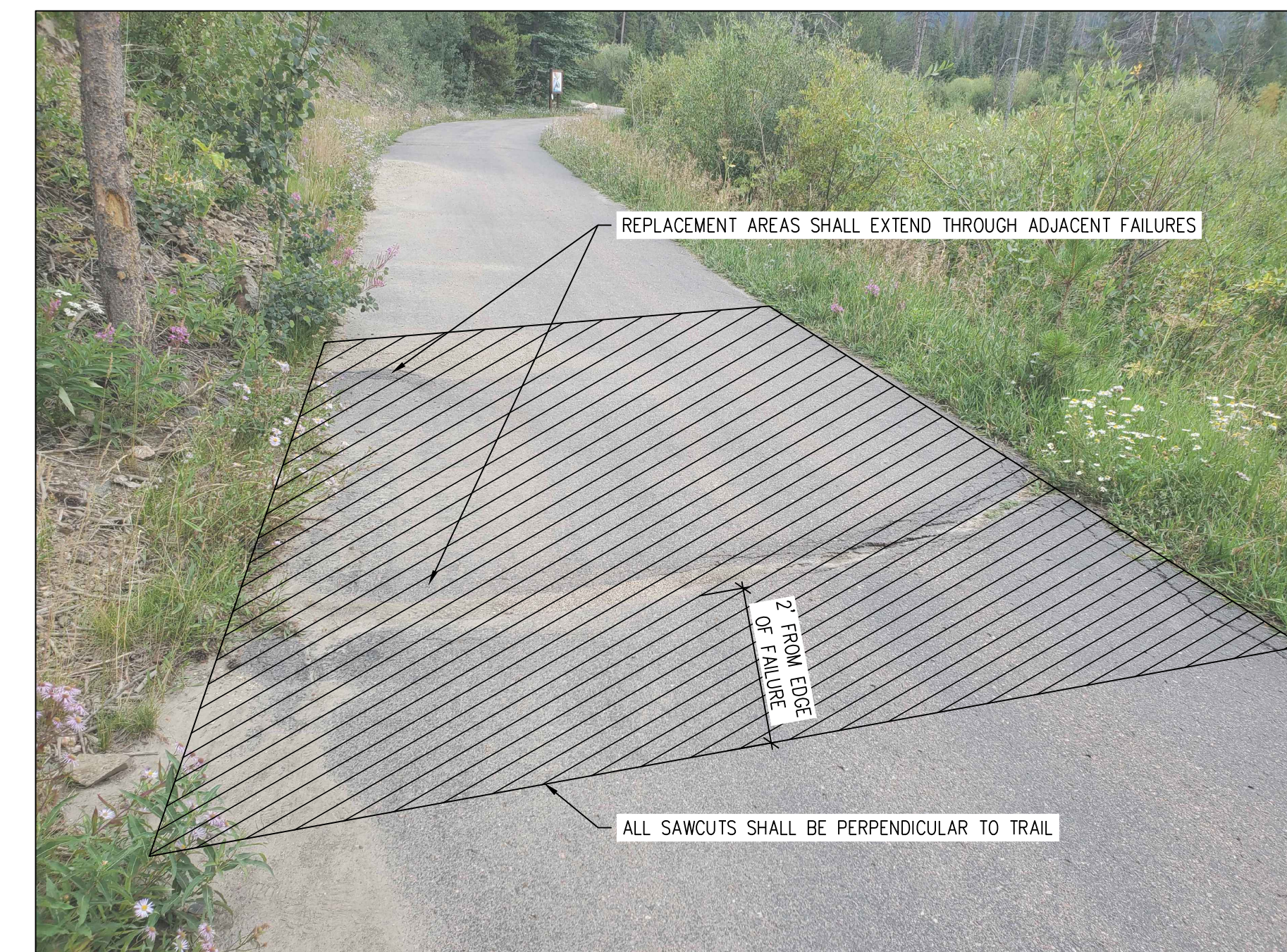
REPRESENTATIVE EXAMPLE OF FAILURE REPLACEMENT AREA
