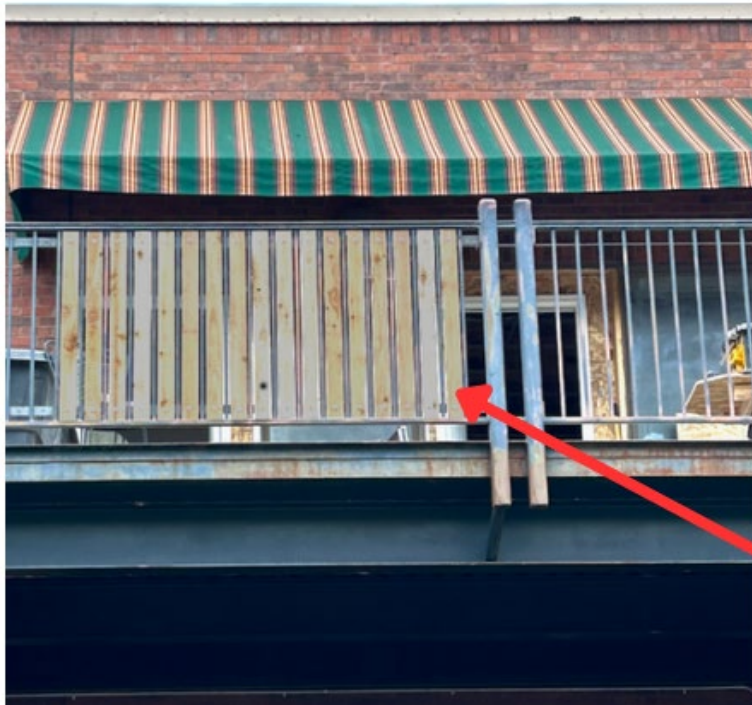
Figure 4 Installed proposed wood slats (to be stained)
