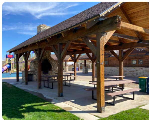
FIGURE 6–33. The shelters at Hideaway Park are consistent in material and scale with the adjacent public restroom.
