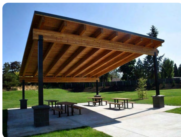
FIGURE 6–35. A modern shade structure provides a contemporary alternative to the rustic aesthetic and allows for snow shed. Image courtesy of Tualatin Hills Parks and Recreation, 2024.
