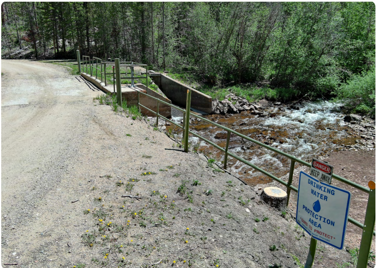
FIGURE 2–67. View of existing infrastructure at the site of Ranch Creek Park.
