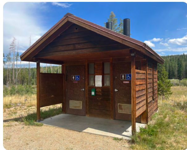
FIGURE 6–31. The vault toilet at St. Louis Creek Campground in the Fraser Valley uses natural materials to match the surrounding aesthetic.
