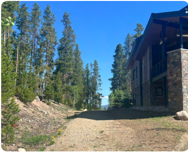
FIGURE 3-9. This HOA trail within the neighborhood passes within 10-feet of a residence without any buffer.
