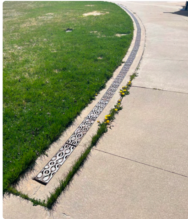
FIGURE 2-10. Decorative trench drain.
