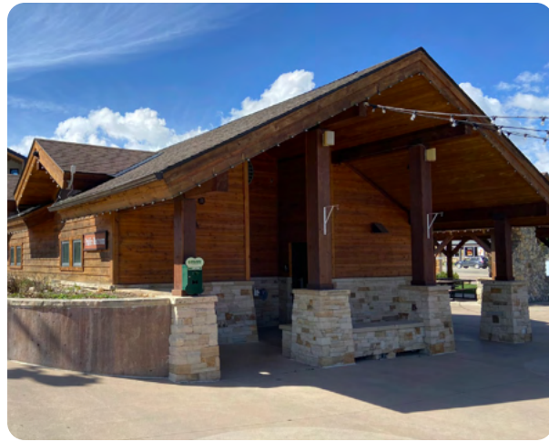
FIGURE 6–27. The public restroom at Hideaway Park provides a rustic appearance with the use of stone and wood materials.
