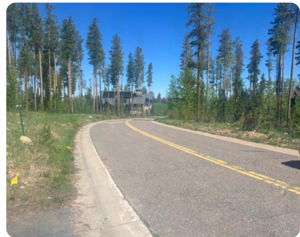
FIGURE 3-14. Some existing trails intersect directly with roads that have no shoulder or location for users to walk. They lack any signage or striping that would indicate an adjoining trail to a vehicle. This presents a hazard to both trail users and vehicle operators.
