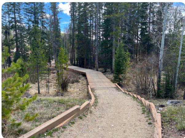
FIGURE 2–24. Boardwalk with retaining walls along the wetland area of Confluence Park.
