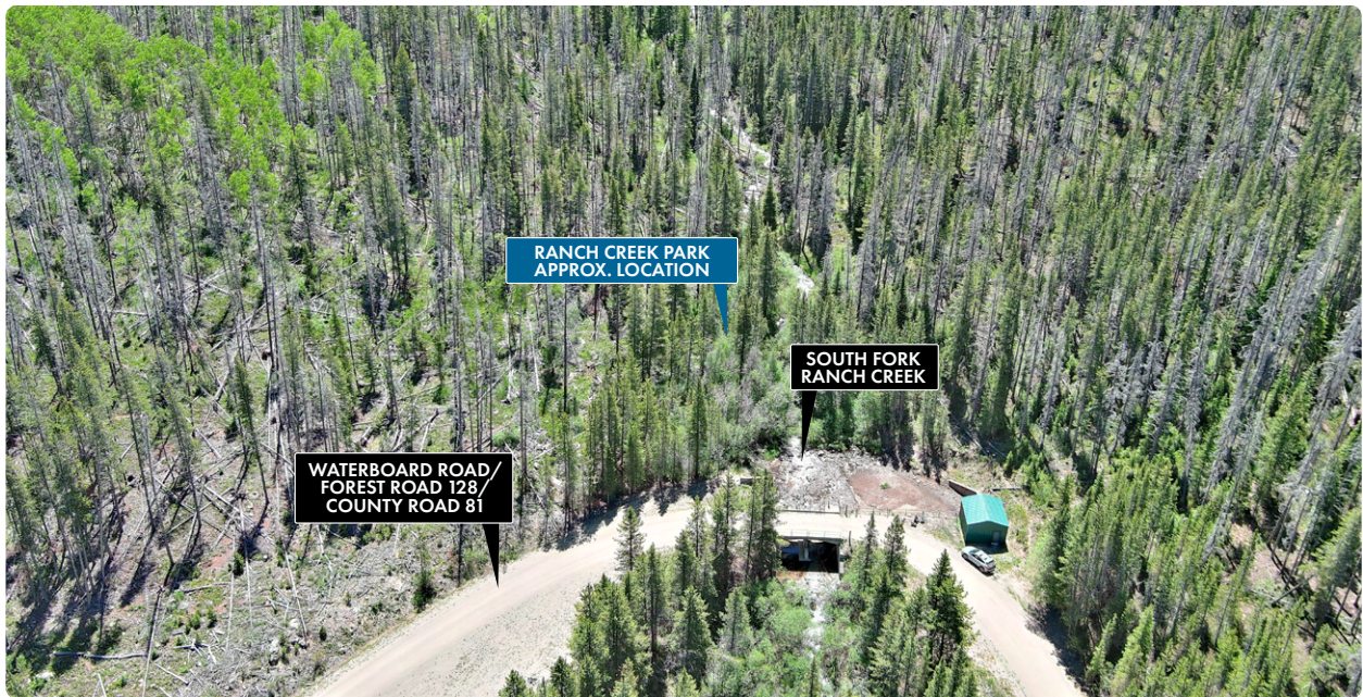
FIGURE 2–65. The future Ranch Creek Park recommended program includes amenities for passive recreation.
