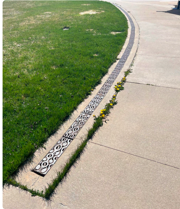
FIGURE 2-10. Decorative trench drain.
