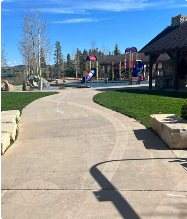
FIGURE 2-9. Etched concrete paving at park entrance.
