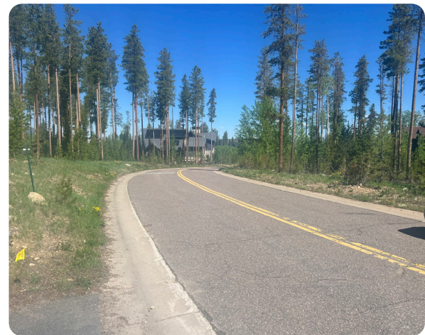
FIGURE 3-14. Some existing trails intersect directly with roads that have no shoulder or location for users to walk. They lack any signage or striping that would indicate an adjoining trail to a vehicle. This presents a hazard to both trail users and vehicle operators.
