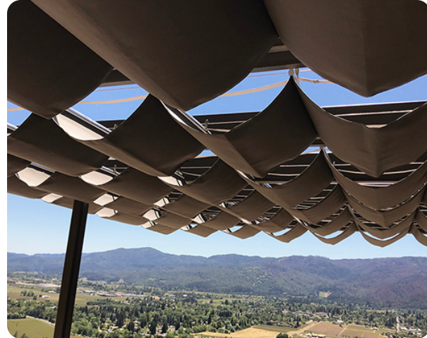
FIGURE 6–36. A retractable fabric shade structure encourages seasonal use and provides flexibility. Image courtesy of Canvas Works, 2023.
