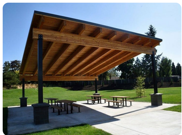
FIGURE 6–35. A modern shade structure provides a contemporary alternative to the rustic aesthetic and allows for snow shed. Image courtesy of Tualatin Hills Parks and Recreation, 2024.
