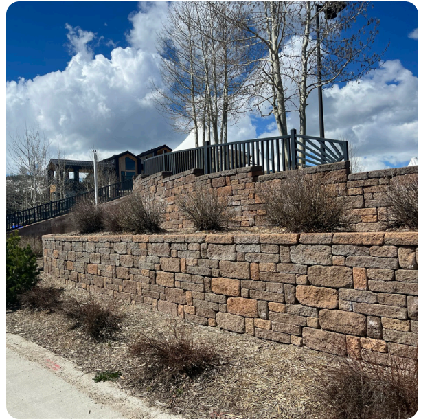
FIGURE 6–39. Retaining walls at Hideaway Park have visually dynamic patterns and textures and are spaced appropriately to allow for intermittent plantings.
