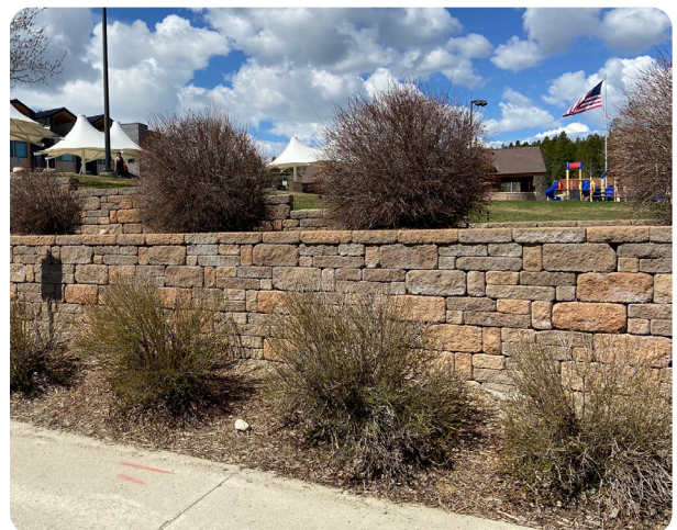
FIGURE 6-9. The shrub installation and spacing at Hideaway Park allows for growth and reducing the risk of overcrowding.
