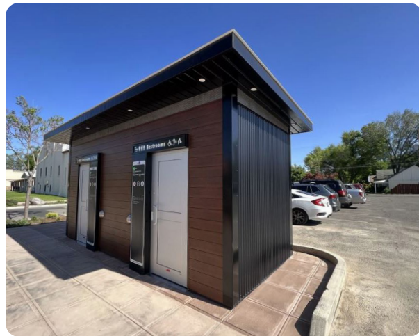
FIGURE 6–28. In the Town of Fruita, this modern, self-cleaning public toilet by UrbenBlu, a Canadian-based company, has proven to be an excellent solution for parks and trailheads.
