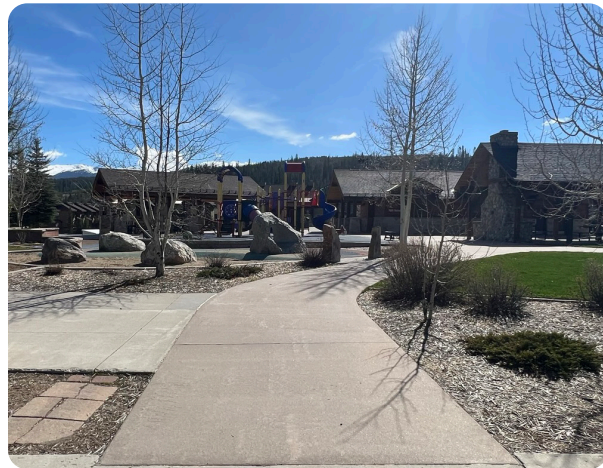
FIGURE 6-1. Example of integral color paving in Hideaway Park.
