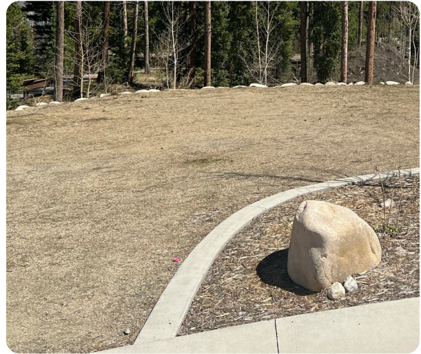
FIGURE 6-2. Existing concrete mow band at Hideaway Park, north of the Rendezvous Event Center.
