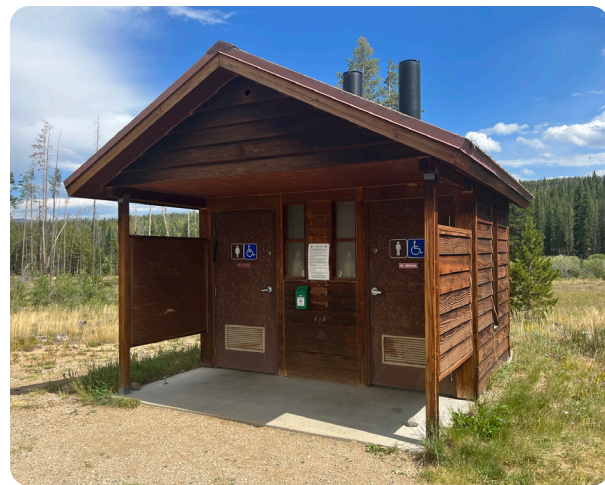
FIGURE 6–31. The vault toilet at St. Louis Creek Campground in the Fraser Valley uses natural materials to match the surrounding aesthetic.
